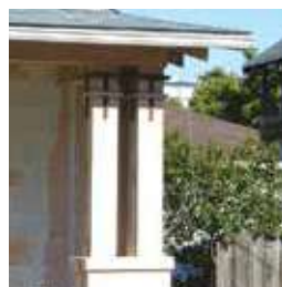
Half-Height Double Post on Pier
