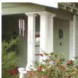
Half-Height Double Post on Pier
