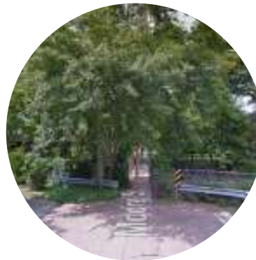
Ward Creek crossing at Moore Street
